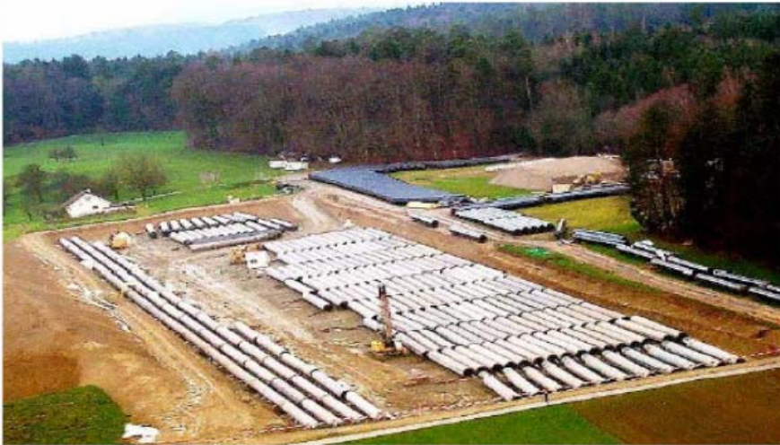
Existing storage technology Buried gas storage near Zurich, Switzerland Operating pressure 1000 PSI
